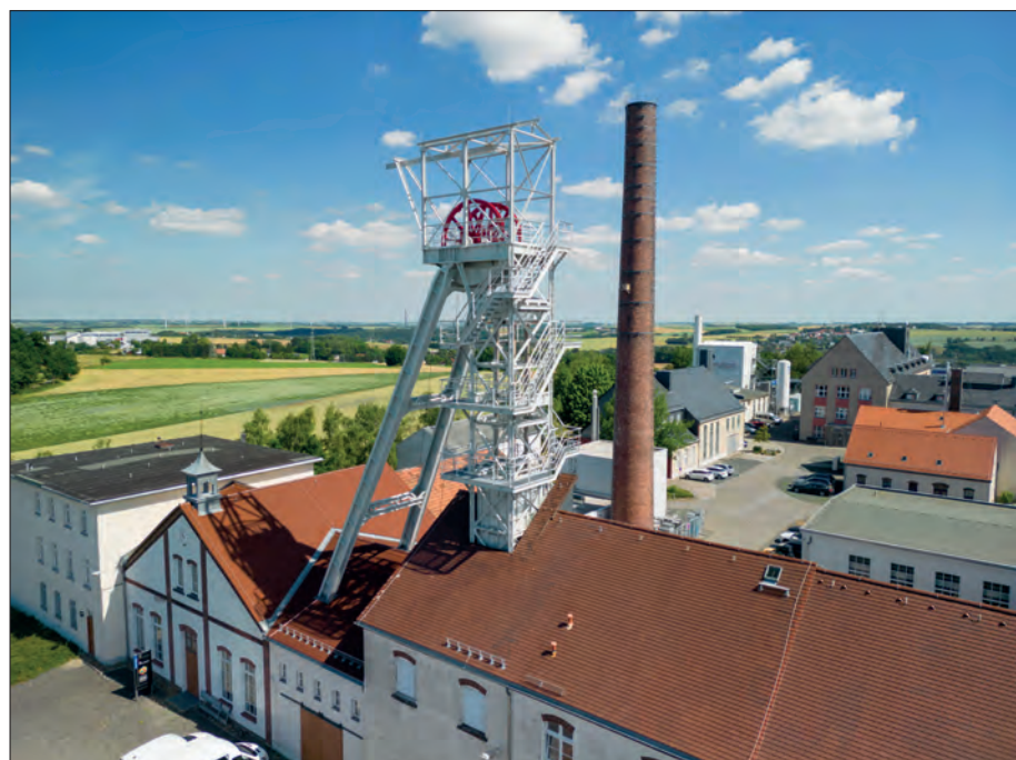
Fig. 1: Shaft tower at the Reiche Zeche shaft (Foto: Jens Kugler).
